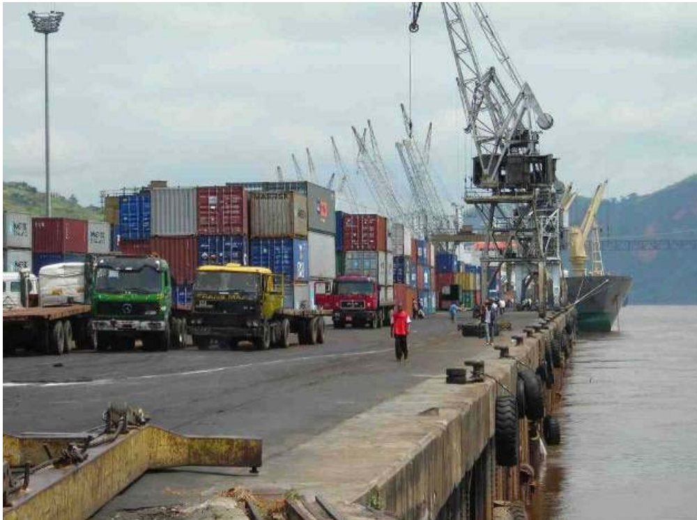
Figure 10-Operational Dock & Crane Area
