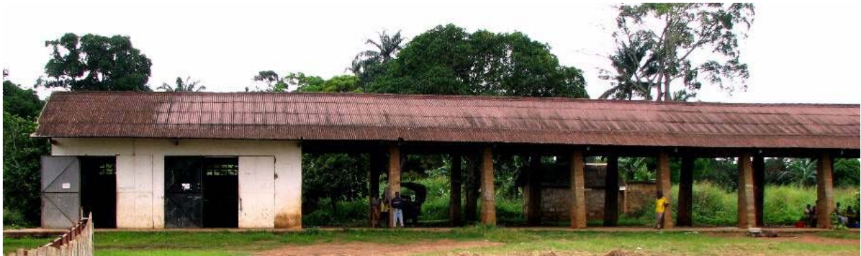
Figure 3 - Location of Generator and Storage Shed
