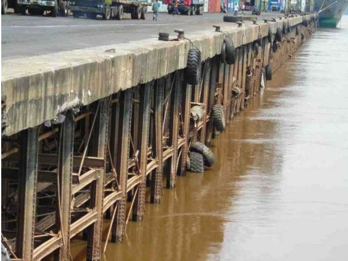
Figure 14 - Operational Dock Pilings
